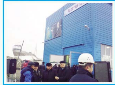
Outside View of Karatal Powerstation in Kazakhstan
