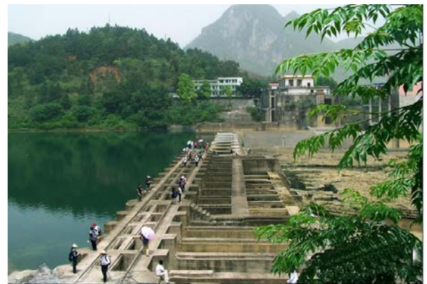
The bulb turbine unit is installed in Nuomintan station in Guangxi Province, China
