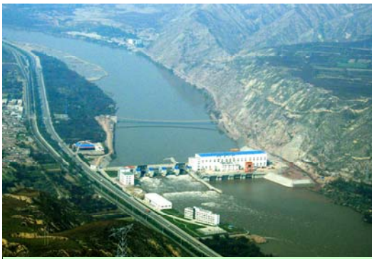
The bulb turbine with second largest runner diameter installed in Chajjiaxia station, Gansu Province, China
