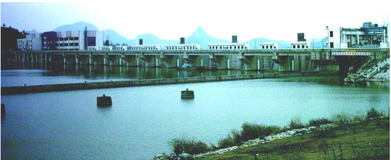
The bulb turbine with runner diameter 5.8m, the largest diameter in China, installed in Mengzhouba station, Shaoguan in 1997. Guangdong
