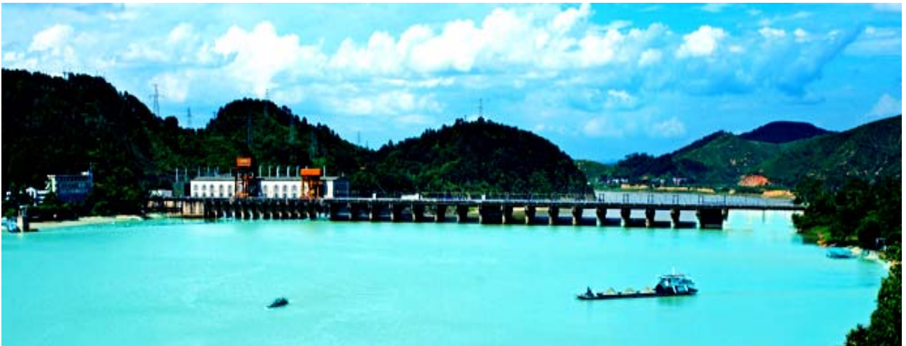
The unit, used in new cooling technology in stator and rotor, installed in Shanxiu, Guanxi Province, China
