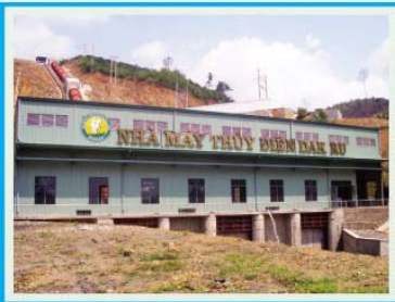
Outside View of Powerstation in Dak Nong of Vietnam
