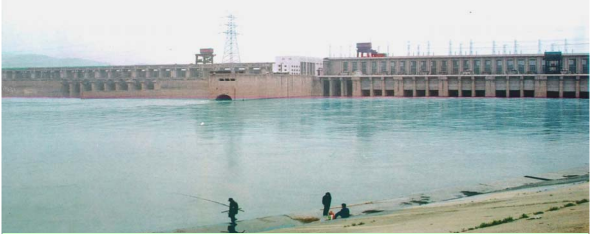
Hydro-generator units installed in the Gezhouba Power Station, China
