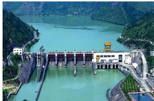
The unit using new cooling technology in stator and rotor installed in Liupu station, Gangxi Province, China
