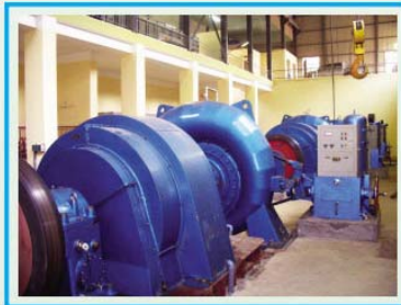
Powerstation with 3x2.5MW Francis Units in Dak Nong of Vietnam
