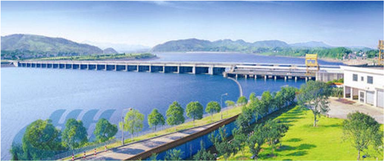
The unit using new ventilation and cooling technology installed in Dayuandu station, Hunan Province, China
