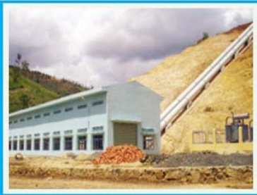
Outside View of Powerstation in Dak Lak of Vietnam
