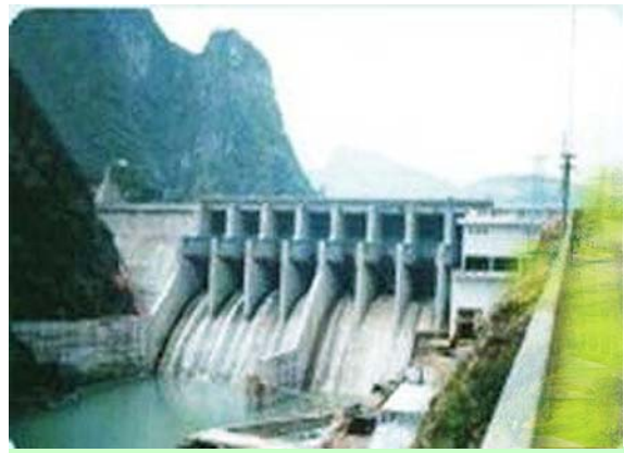
The unit is installed in Yutang station, Zhangjiajie (World Natural Heritage), Hunan Province, China
